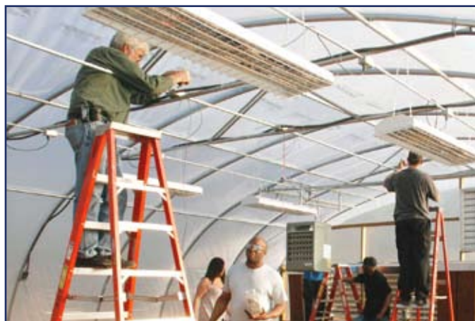
Rockingham Community College students provide electrical wiring to a greenhouse owned by a local non-profit.
